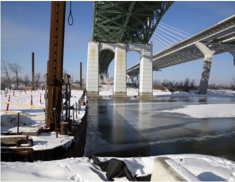
Pier 1E surrounded by a jetty for the deconstruction of the east cantilever span
